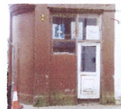
12 Cross St unoccupied more than five years
